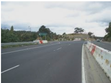
1 st Left Turn at top of Tunnel Hill
